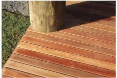
**Description:** An Australian hardwood used throughout NZ as telegraph poles. Extremely durable heartwood is used for interior and exterior beams and now commonly used for decking, cladding and outdoor furniture.
